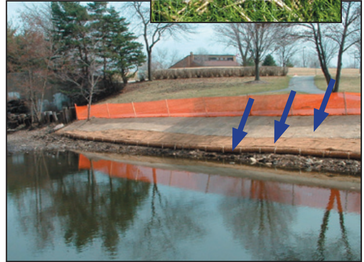
Shown here are different types of RECPs and coir fiber roll being used to stabilize the shoreline.
